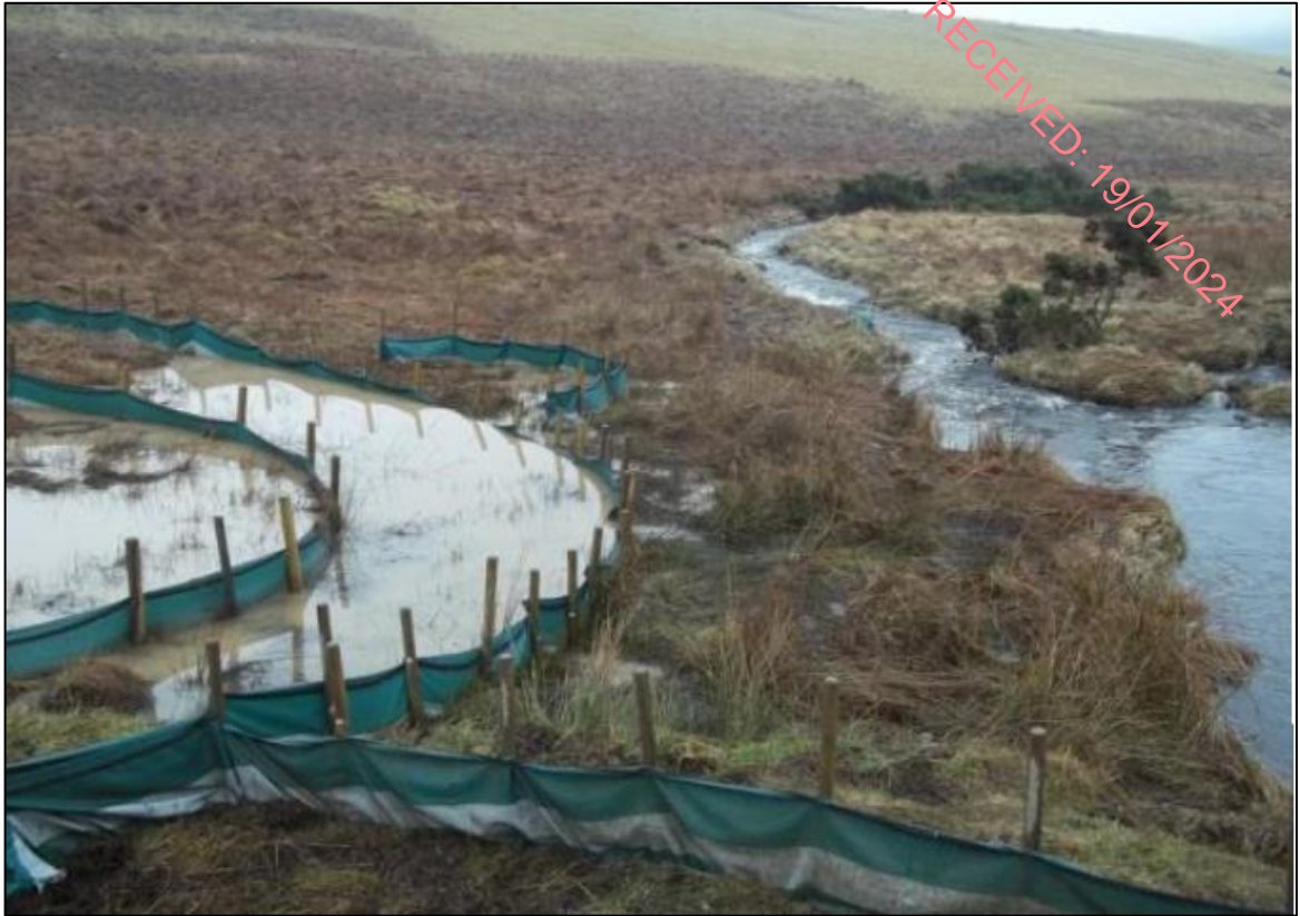
Plate 5.2: Photograph of silt fencing
