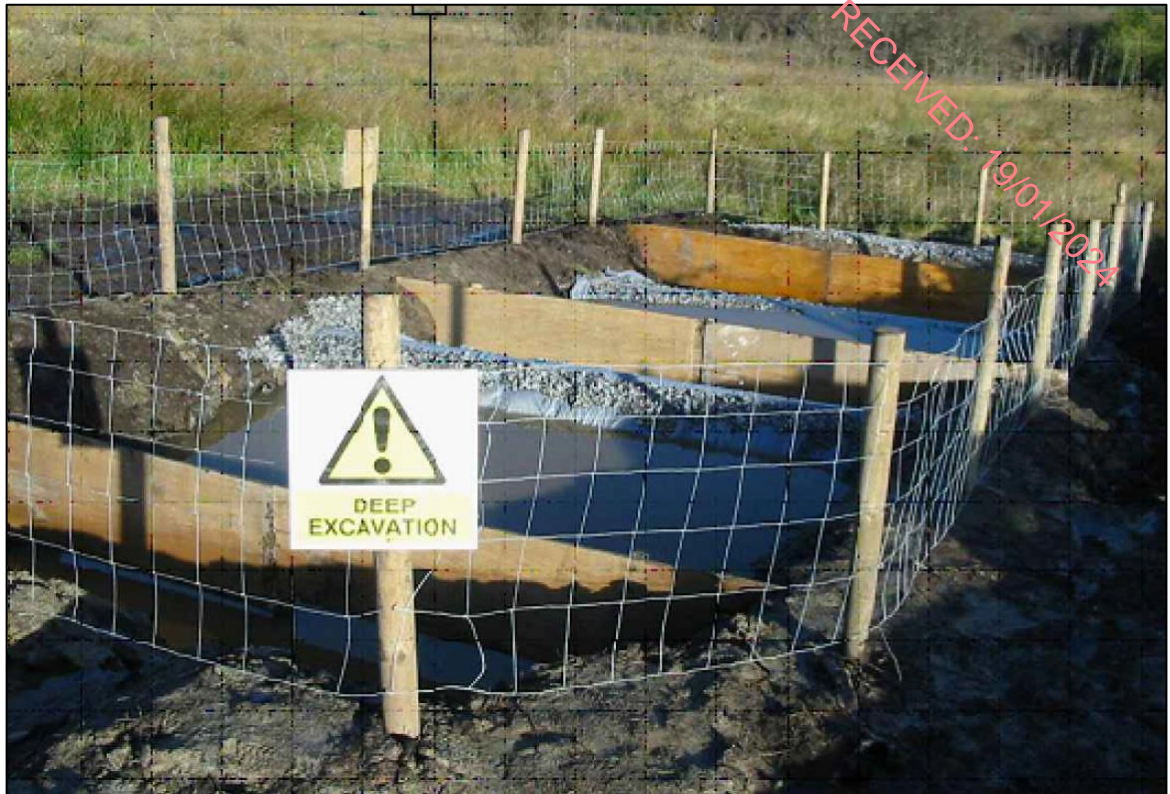
Plate 5.4a: Completed settlement pond system
